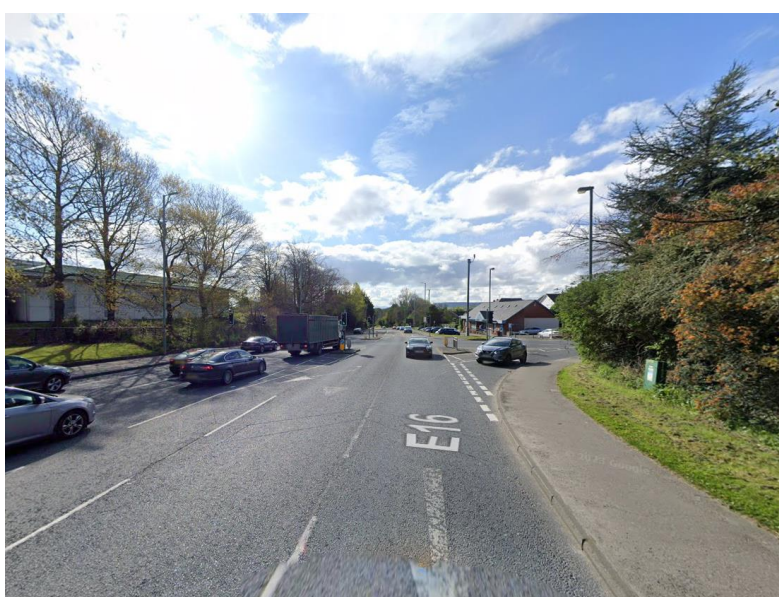
Figure 2: A6 junction with Belt Rd (Photo source: Google Earth - taken Apr 2023)
